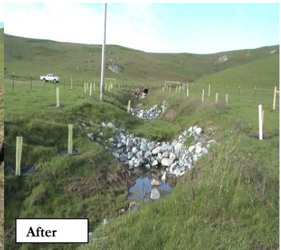
Gully repair using loose rock checks
