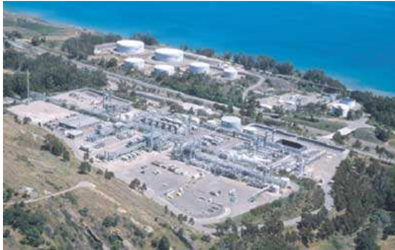
Figure 3 Gaviota Oil Heating Facility (foreground) Gaviota Oil Terminal (background, since removed) (Source: SBCO P&D Energy Division Website)
