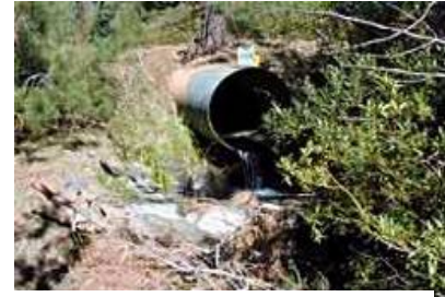
Figure 3.9: Perched pipe
