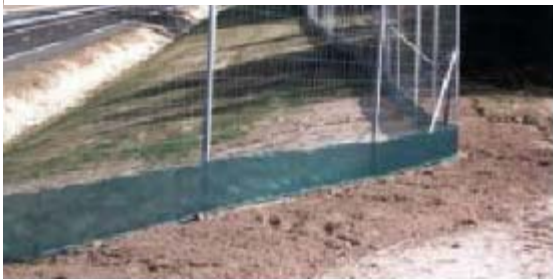
Figure 3.7: Wide mesh chain link fence for large mammals, with a fine mesh fence border for small mammals and amphibians
