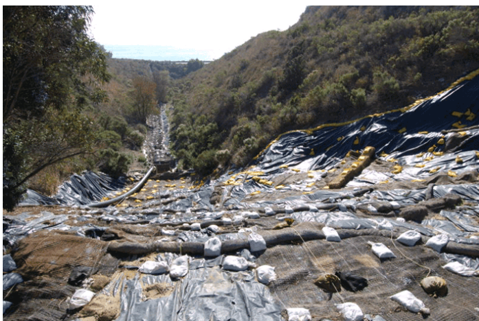
Fill Pad Slope
