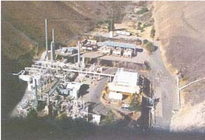
Hercules Gas Plant in 1989
