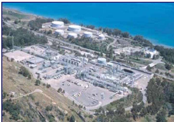
Gaviota Oil Heating Facility (GOHF) in foreground (mountain-side of Hwy 101) GTC's Gaviota Terminal is in background (ocean-side of Hwy 101)
