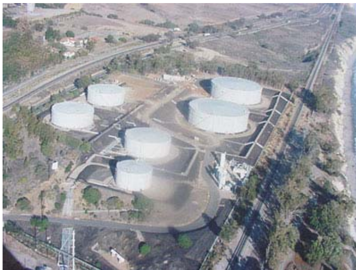
Prior to demolition
