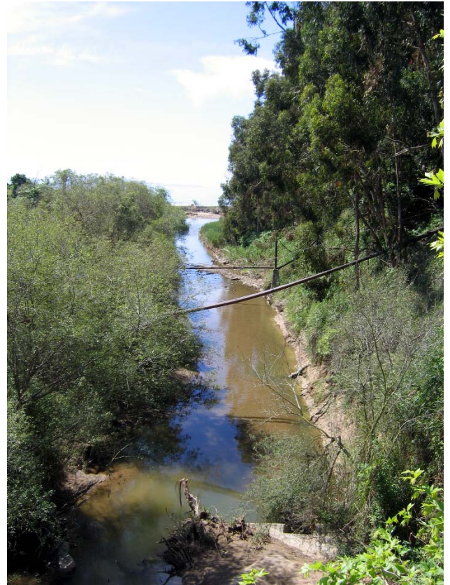
Bell Creek Crossing
