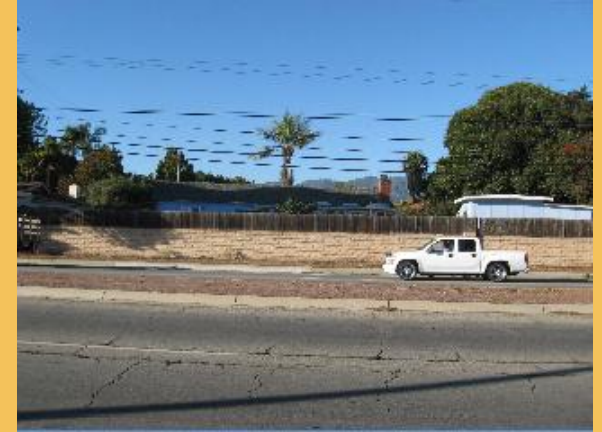
Hollister Ave Wall - North
