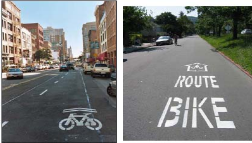
Figure 4.7-2: Examples of Bicycle Boulevard Pavement Markings
